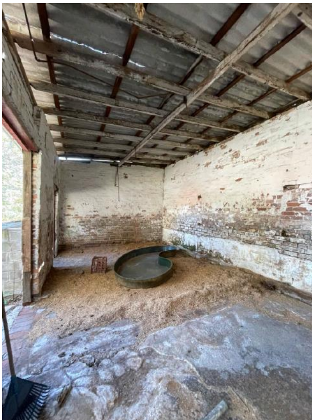
Figure 18: Interior of stable block
