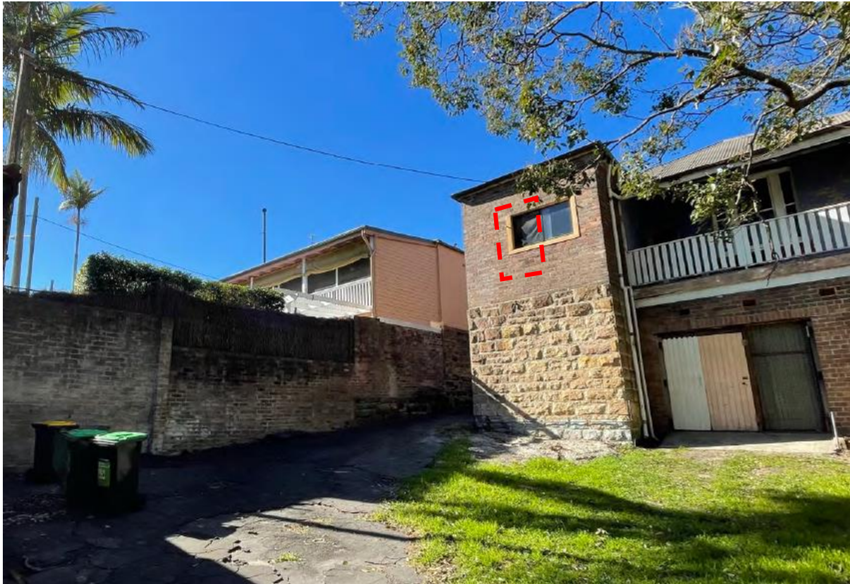
Figure 57: Rear of existing building (Dwelling 1) and neighbouring site (3 Victoria Road) as viewed from backyard, looking south-east. New approx. size and location of W07 shown in red dash
