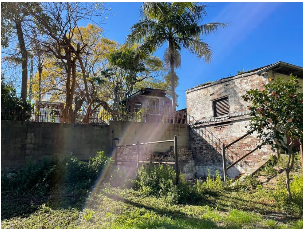
Figure 20: Rear of stable block, view east to 1 Alexandra Lane
