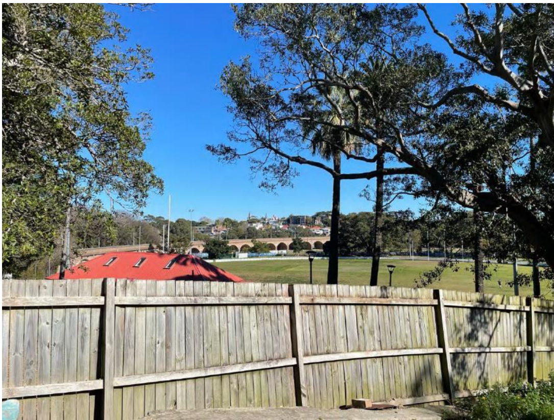
Figure 14: View west across Jubilee Oval and Jubilee Park viaduct, as viewed from the site's south-western boundary
