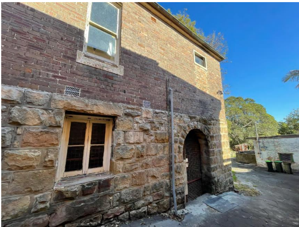
Figure 12: Existing sandstone base, proposed to be used as lower ground level art studio that can also function as a separate, self-contained dwelling – new timber framed stained glass window proposed to arch
